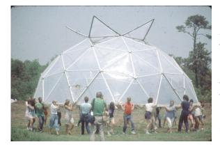
When the I pillows are inflated, the entire dome is put under compressive load that tends to oppose the considerable wind lift, This preloading, together with the anchoring provided by buried concrete blocks tied to the lowest hubs, has withstood 30 inches of snow load and winds well above 100 mph. This may be considered good performance from a structure that weighs but 1/2 lb/ft2 of floorspace (less than 500 lbs total). The light weight not only results in low shipping
