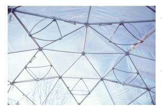
The physical performance has been good. The biological performance has equaled the original New Alchemy Ark in output per square foot, that is, commercial production quantities. Moreover, the pillow dome's natural air circulation patterns have eliminated the need for that nuclear fan. The dome also casts but 1/5th the shadow of a more conventional greenhouse, important for winter growing.
